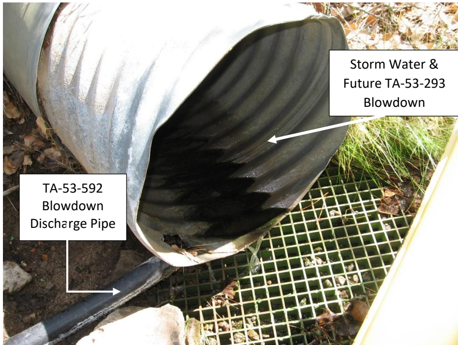
Photograph - NPDES-03A113-18-002 Outfall 03A113 Condition at Discharge Location
